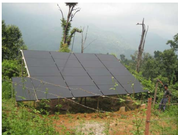
Solar panels used for water lifting in Bimrekhola, Risku VDC, Udayapur District
