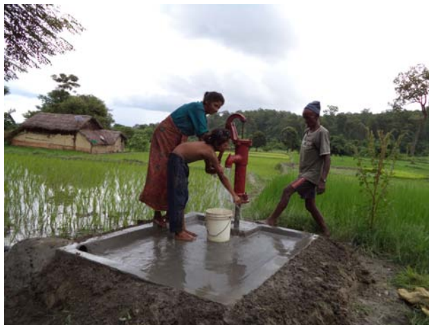
Tube well rehabilitated with a platform in Bagauda VDC, Chitwan District
